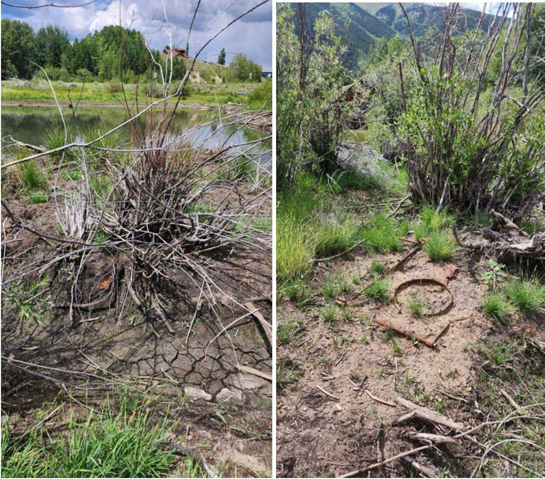
Figure 19. Photos of scrap buried in the downstream embankment of the Barn Pond.
