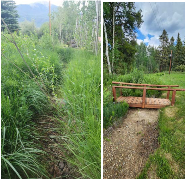
Figure 9. Area 1 U shaped ditch just down ditch of the “West Fork Split”
