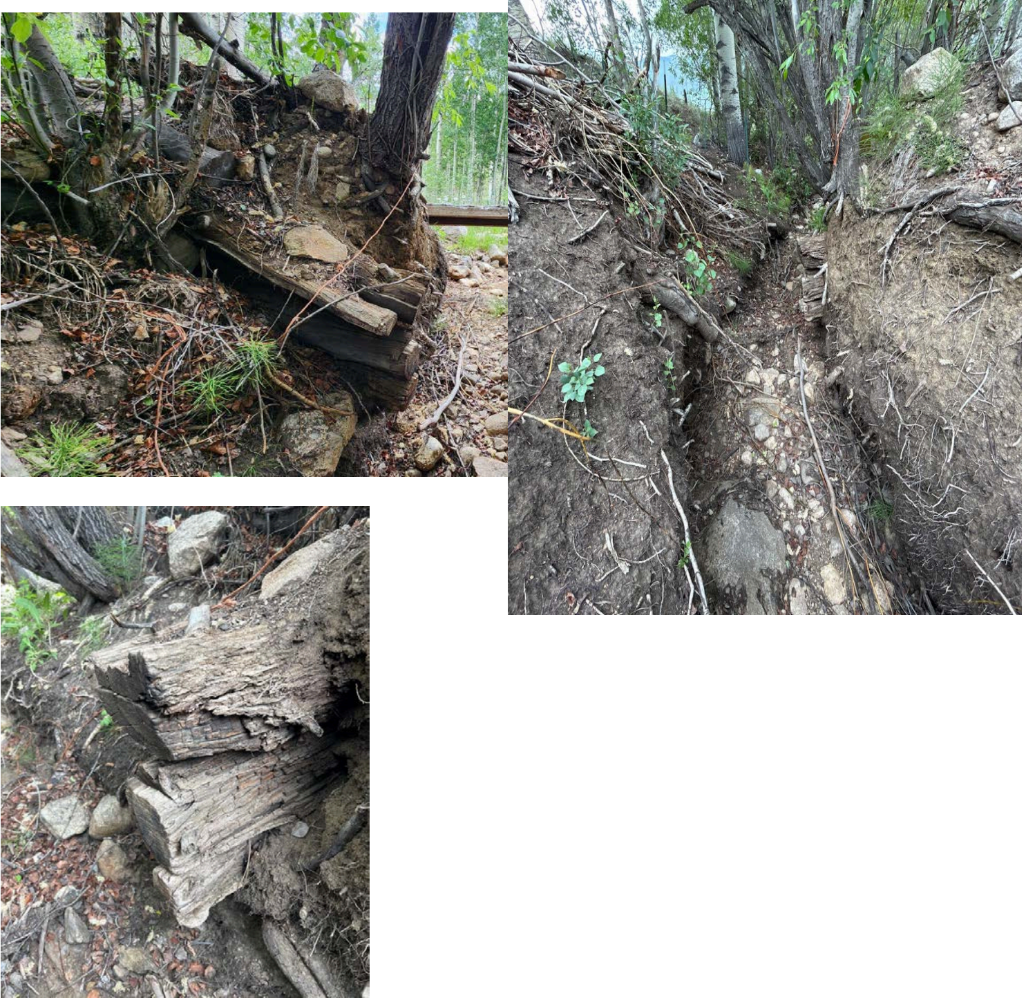
Figure 13. Area 3 photos of excavated cut through “glacial moraine”.
